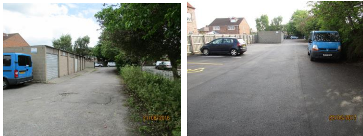
Re-surfaced and enlarged car park.
